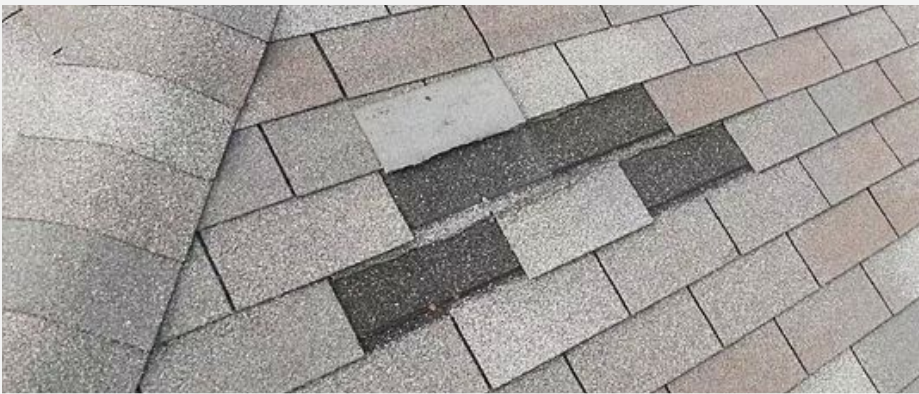
MISSING SHINGLES
